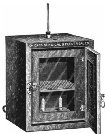
Fig. 410. The Electric Incubator I use for fermenting yeast and urin mixtures. This is accurate to within a small fraction of a degree.
