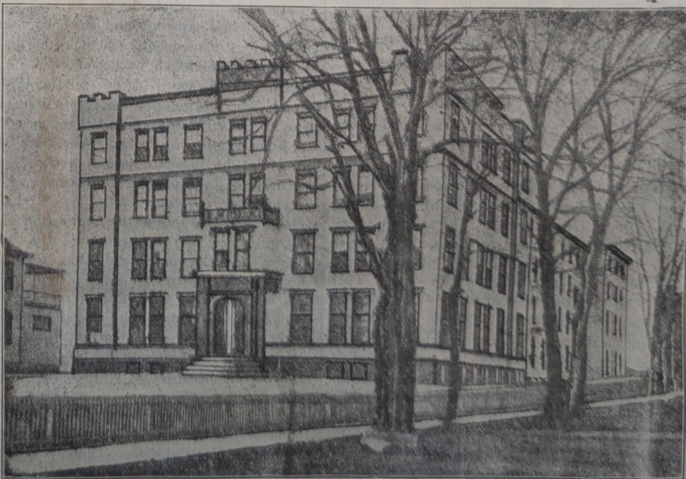
CONWAY HALL, DICKINSON COLLEGE, CARLISLE, PA. (Erected 1905.)
