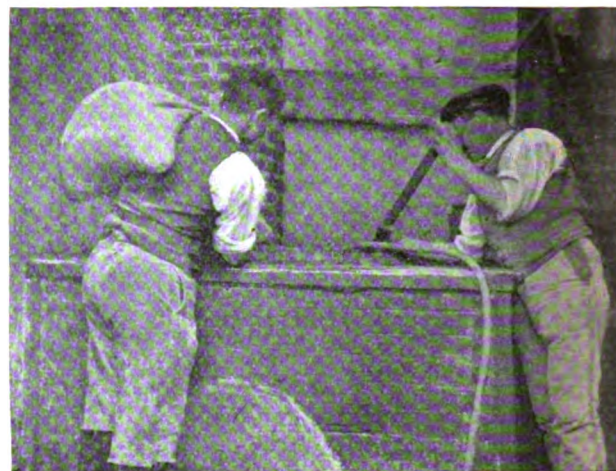
Emptying uranite powder into a caldron.—The first act of purifying
