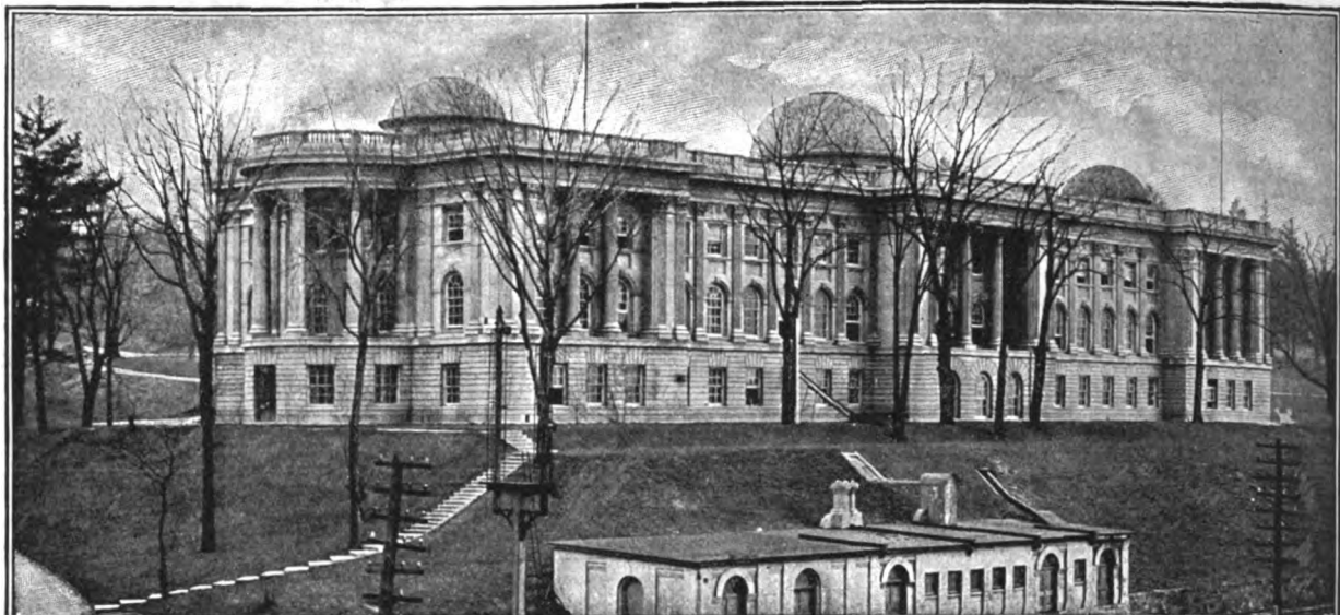
BUILDING ERRECTED AT IRVINGTON ON THE HUDSON FOR THE COSMOPOLITAN MAGAZINE AND THE TWENTIETH CENTURY HOME. The Cosmopolitan Magazine was a pioneer in the experiment of choosing one of the most beautiful places on the Hudson upon which to erect an ideal factory building, moving out from New York, and thus bringing its considerable force of employes into an environment of the most favorable character. This move was regarded at the time as almost equally radical with that of cutting the price of a 25-cent magazine in half—in which the Cosmopolitan was also the pioneer. It may be interesting to the general public to know that both of these moves have proven completely successful.
