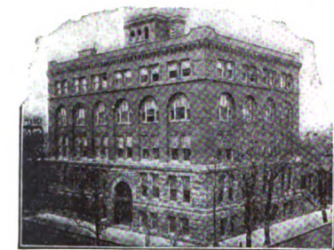
MACHINERY HALL, ARMOUR INSTITUTE OF TECHNOLOGY
