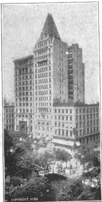
THE HOME LIFE BUILDING, 256-257 Broadway, New York. Our offices occupy sixteen rooms on the fifth and sixth floors, overlooking City Hall Park, the Post-office, and Brooklyn Bridge.
