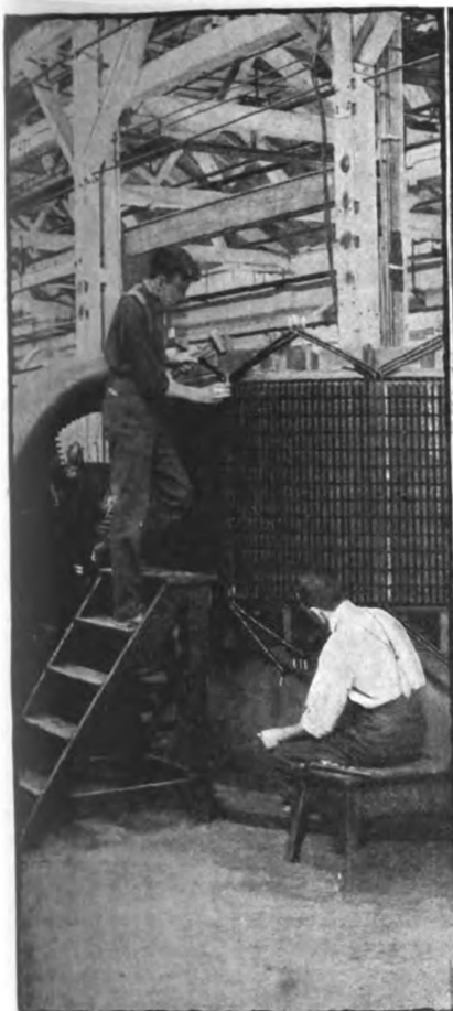
Winding a powerful armature for use at Niagara
