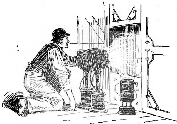
Inside the "furnace"
