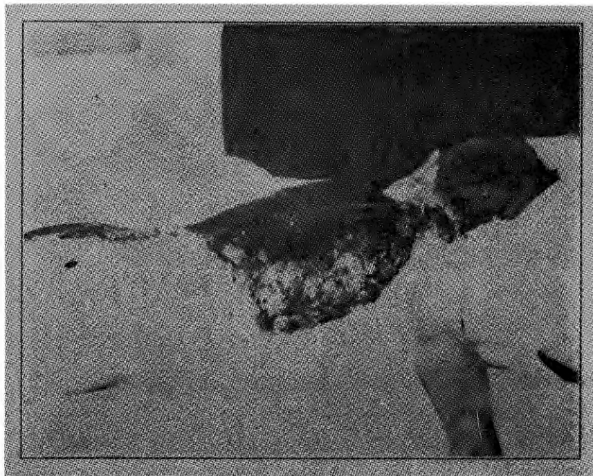
BACK VIEW OF BURNT AREA
