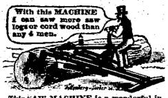
This SAW MACHINE is a wonderful invention. The weight of the man who is sawing does one-half of the work. It saws logs of any size, and will saw off a 2 foot log in 2 minutes. Circulars free. Address. Wns. GILES, Box 538, Cincinnati, Ohio.
