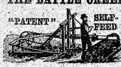
To calculated f a two or more horses; adapted to any power with belt or tumb in rod. Ligat draft and early handled. Will cut from 30 to 57 cords stove wood per day. Also, OlROULAR WOOD MILLS for long or show wood. Power much improved this sesson. Manufactured and sold with or without power by the BATTLE CREEK MACHINERY CO. Battle Creek, Mich. ET Sent for Circular and Price-List.
