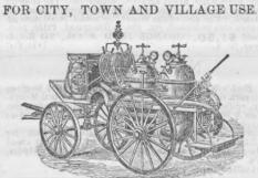
It is more effective than the Steam Fire Engine, because it is instantaneously ready and throws a powerful stream of carbonic acid, gas and water for any length of
