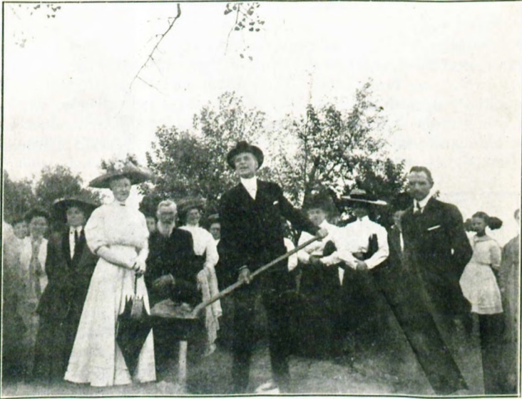
THE PASTOR TURNING THE FIRST SHOVEL OF DIRT.
