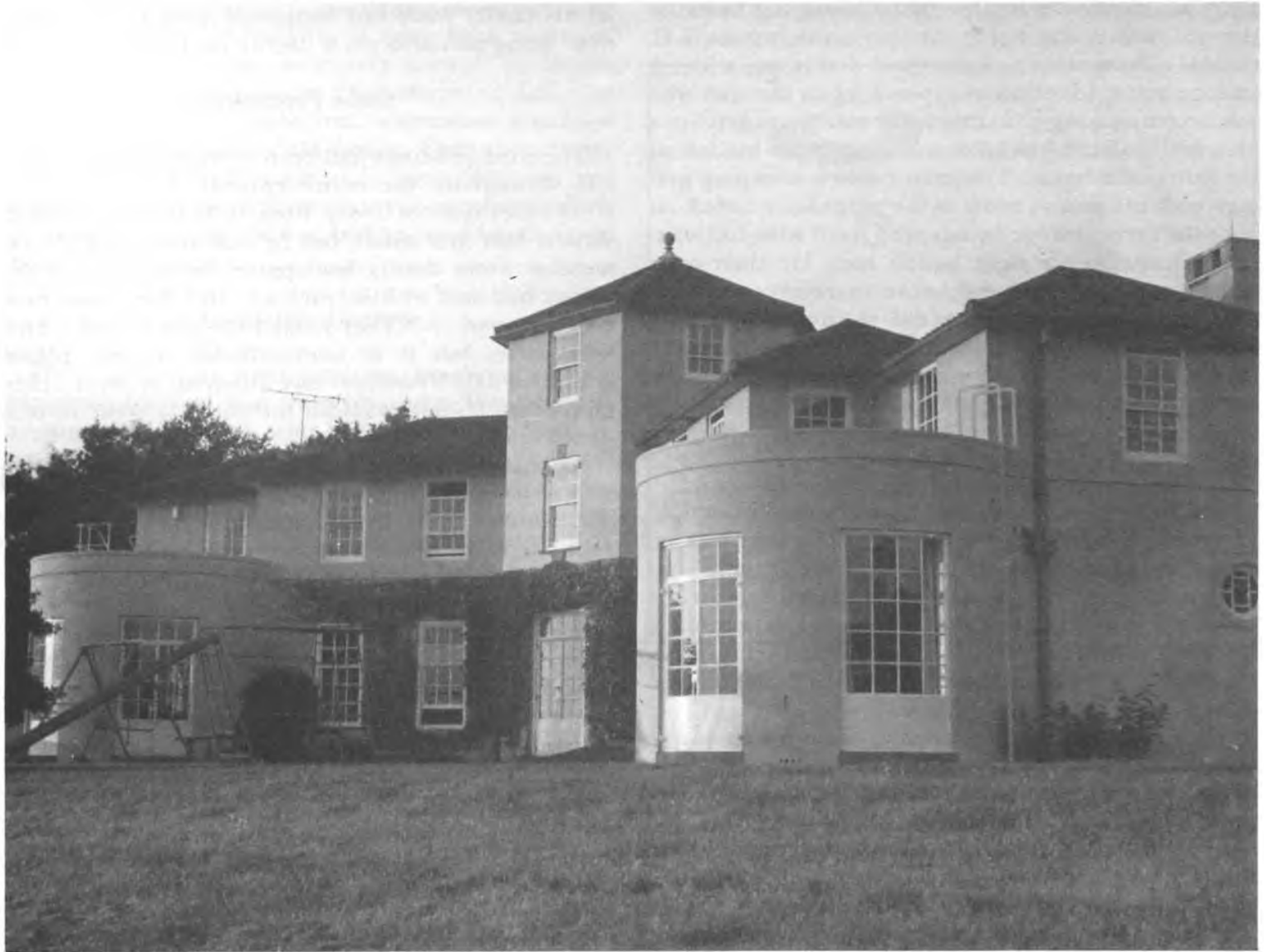
High Hurlands Hospital, Passfield, Hants. Door centre, where entity appeared.
