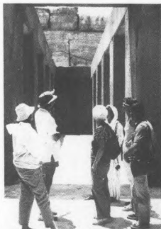
Fig. 8. Temple near the Sphinx has an envelope, or skim, of polished granite blocks over an older limestone core.
