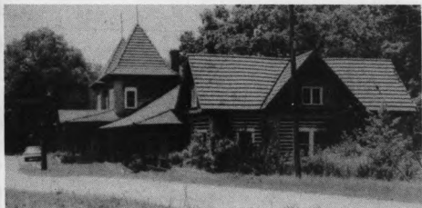
The Oklahoma, the other luxury hotel, still stood in 1962 when this picture was taken. It later burned. Rustic log construction, red tile roofs and spacious fireplaces were features of Harvey's buildings.
