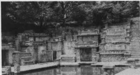
Grecian-style amphitheater said to seat 1000 persons faced the speaker's platform in the lagoon. It was built of native stone and concrete.
