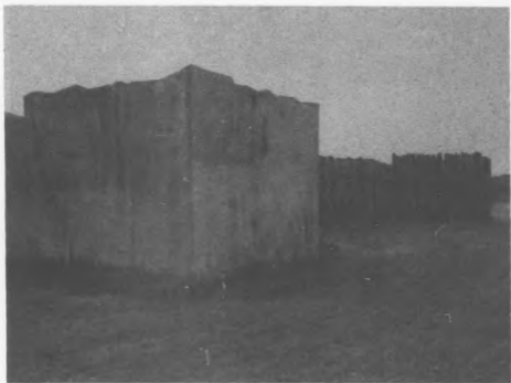
The great wall, at least 7800 feet in length, was built of heavy timbers 20 feet long and plastered with clay to protect against fire arrows, insects and weathering.
