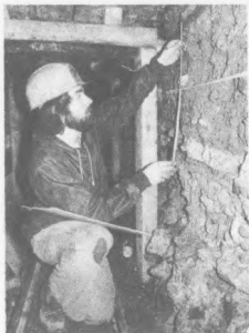
All along telephone tunnel more than 200 yards long, massive basilica and courtyard floors form tunnel walls and roof.
