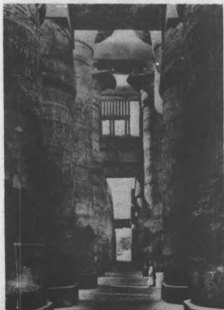
Forest of 134 gigantic columns supports ceiling of hypostyle hall. Columns in two central rows are 64 feet high; circumference of each is 33 feet. These are not monolithic blocks of stone but are made of half-drums which could be moved relatively easily.
