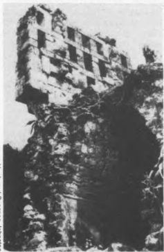
Photo of northeast corbeled room shows mask support of front of roof comb which originally supported stucco human figure.
