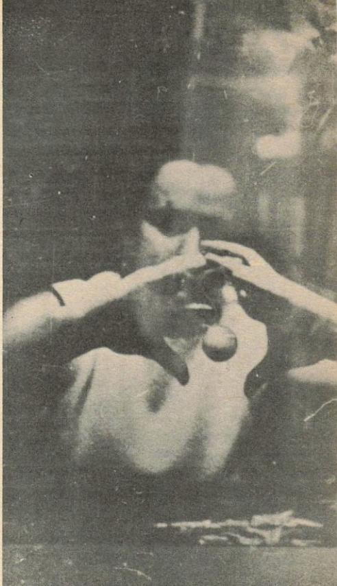
The biometer consists of two electrodes, an outer zinc cylinder and an inner copper rod, separated by dielectric material and connected by insulated flexible wires to a measuring device. The experimenter presses the cylinder into the subject's hand and completes the circuit by pressing his other hand onto the subject's body. An electrode is used at the point of the device to probe the skin. The indicator needle of the micrometer deflects when an acu-
