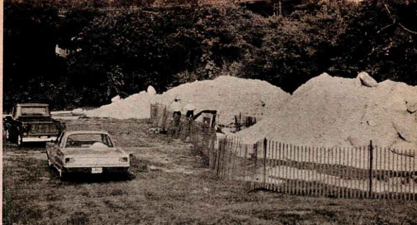
After experts had concluded, "No major sources of water are available," Jim Kidd's findings led to large-scale well-drilling operation which produced 2,000,000 gallons a week. Pump visible here, with capacity of 500 gallons a minute, was employed to keep holes dry enough so digging could proceed.
