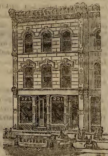
Front view of the CARPENTER DONATION, a fine, stone front building No. 221 West Madison St., Chicago, now occupied by the National Christian Association. The fee simple will be given by Mr. Carpenter if other friends raise $30,000 by Apr. 1st 1878, in cash or "good, negotiable, interest-bearing notes" to establish a Publishing House and headquarters of the reform. Send donations to the Treasurer at 18 Wabash Ave., Chicago.
