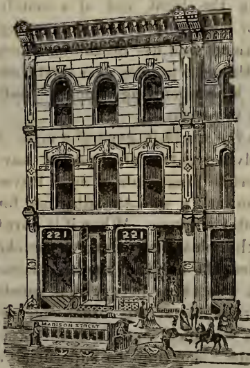
Front view of the CARPENTER DONATION, a fine, stone front building No. 221 West Madison St., Chicago, now occupied by the National Christian Association. The fee simple will be given by Mr. Carpenter if other friends raise $30,000 by Apr. 1st 1878, in cash or "good, negotiable, interest-bearing notes" to establish a Publishing House and headquarters of the reform. Send donations to the Treasurer at 13 Wabash Ave., Chicago.
