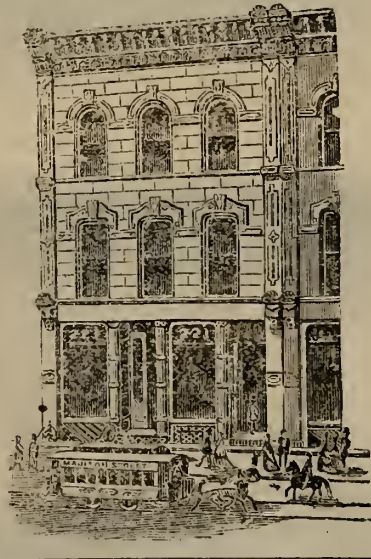
Front view of the CARPENTER DONATION, a fine, stone front building No. 221 West Madison St., Chicago, now occupied by the National Christian Association. The fee simple will be given by Mr. Carpenter if other friends raise $30,000 by Apr. 1st 1878, in cash or "good, negotiable, interest-bearing notes" to establish a Publishing House and headquarters of the reform. Send donations to the Treasurer at 13 Wabash Ave., Chicago.
