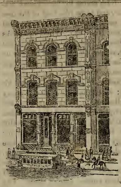
Front view of the CARPENTER DONATION, a fine, stone front building No. 221 West Madison St., Chicago, now occupied by the National Christian Association. The fee simple will be given by Mr. Carpenter if other friends raise $30,000 by Apr 1st 1878, in cash or "good, negotiable, interest-bearing notes" to establish a Publishing House and headquarters of the reform. Send donations to the Treasurer at 13 Wabash Ave., Chicago.
