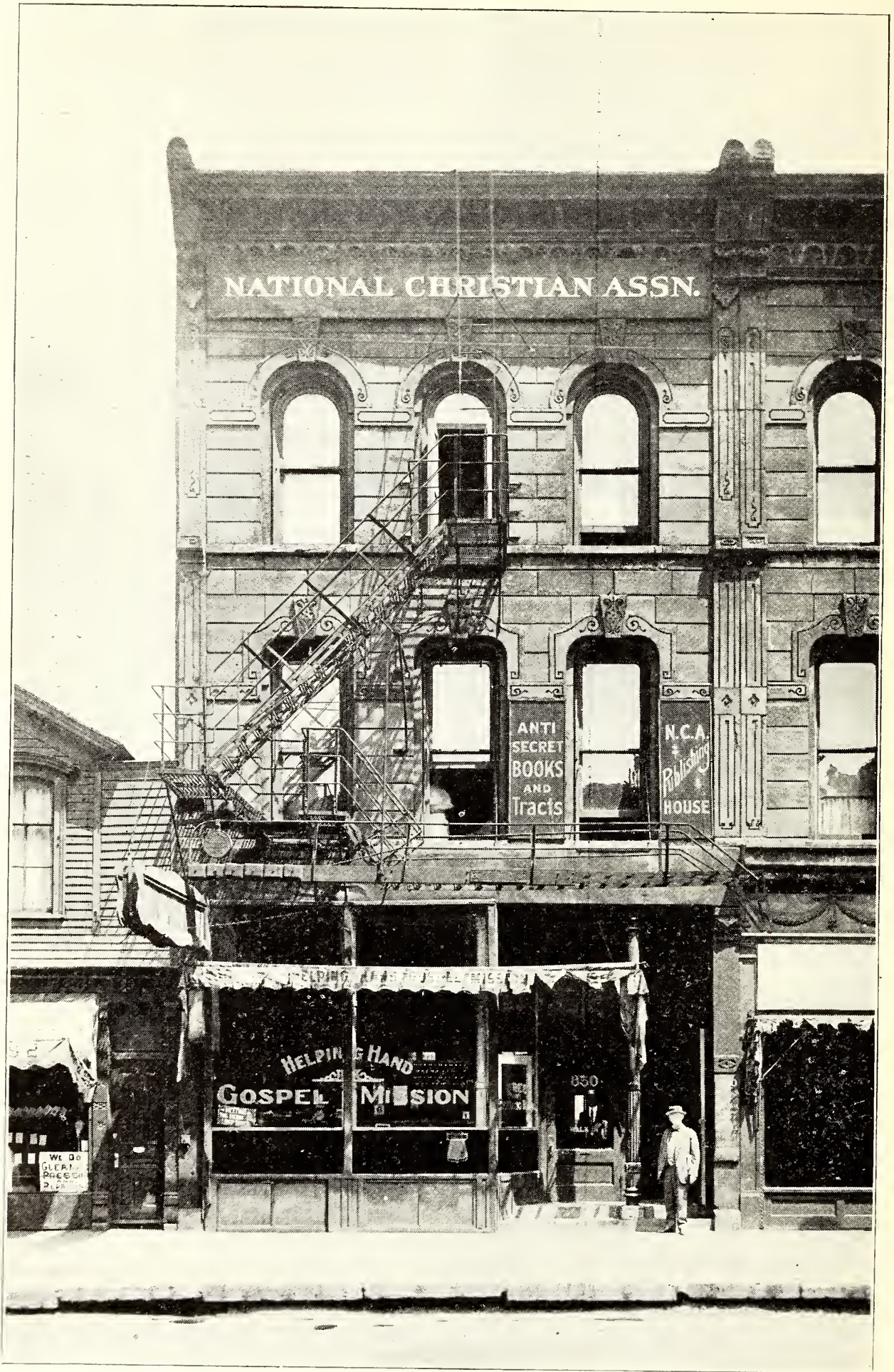
"THE CARPENTER BUILDING."
