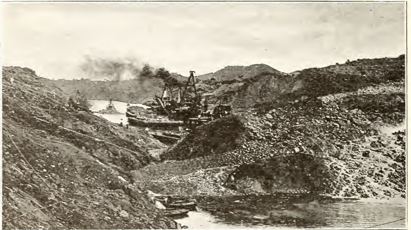
THE CANAL SLIDE, NOV. 3, 1915, COMPLETELY FILLING THE CANAL.
