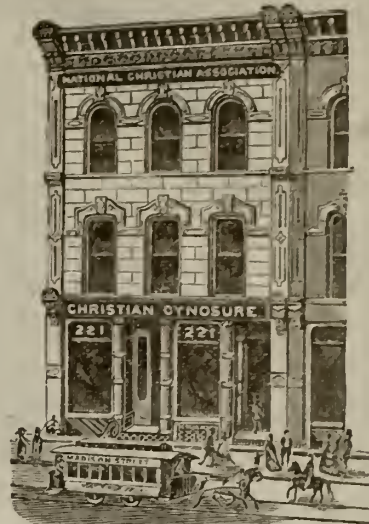
THE N. C. A. BUILDING (The gift of Philo Carpenter.)
