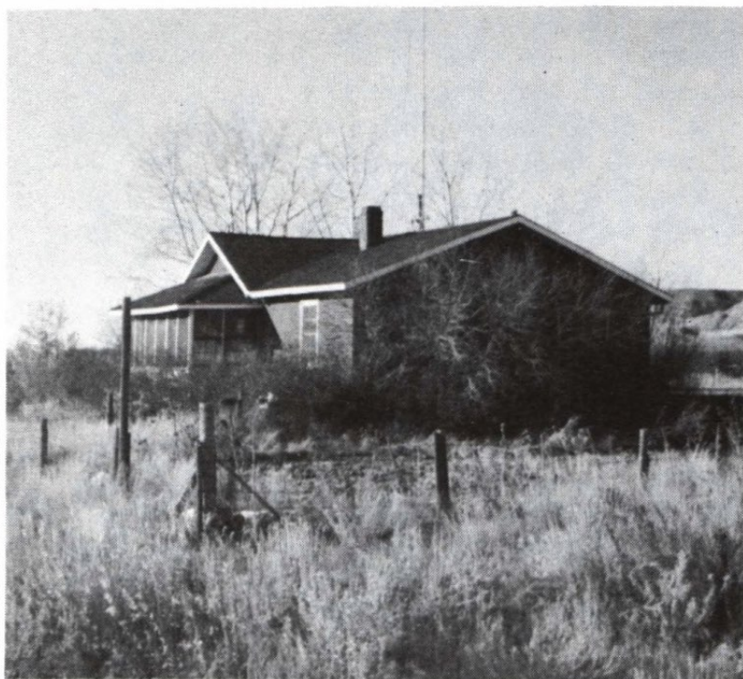
Clappison house seen from landing area.
