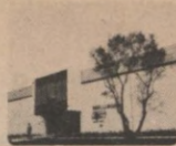
This giant building, new headquarters of I.T.
